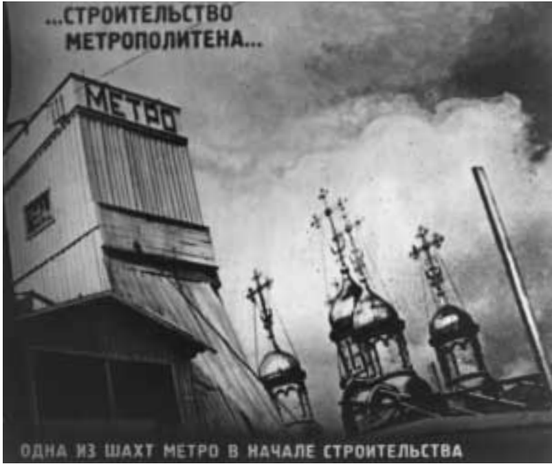
FIG. 3 This slide, part of a slide show on the reconstruction of Moscow for Soviet school children in the 1930s, shows a metro shaft in the beginning of construction. (Soviet slide picture show on the reconstruction of Moscow, box 1, John L. Iliff Collection, Hoover Institution Archives.)
